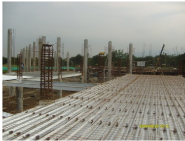
Losa still deck
