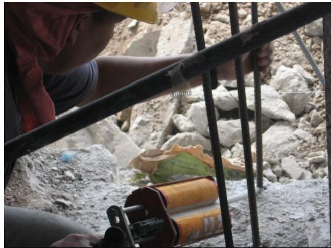
FIGURA 10. APLICANDO ADHESIVO EPOXICO
