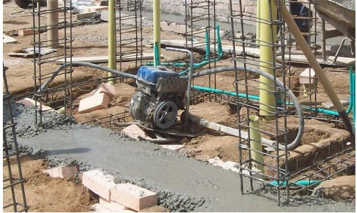
**Figura No. 34: Vibrador**
