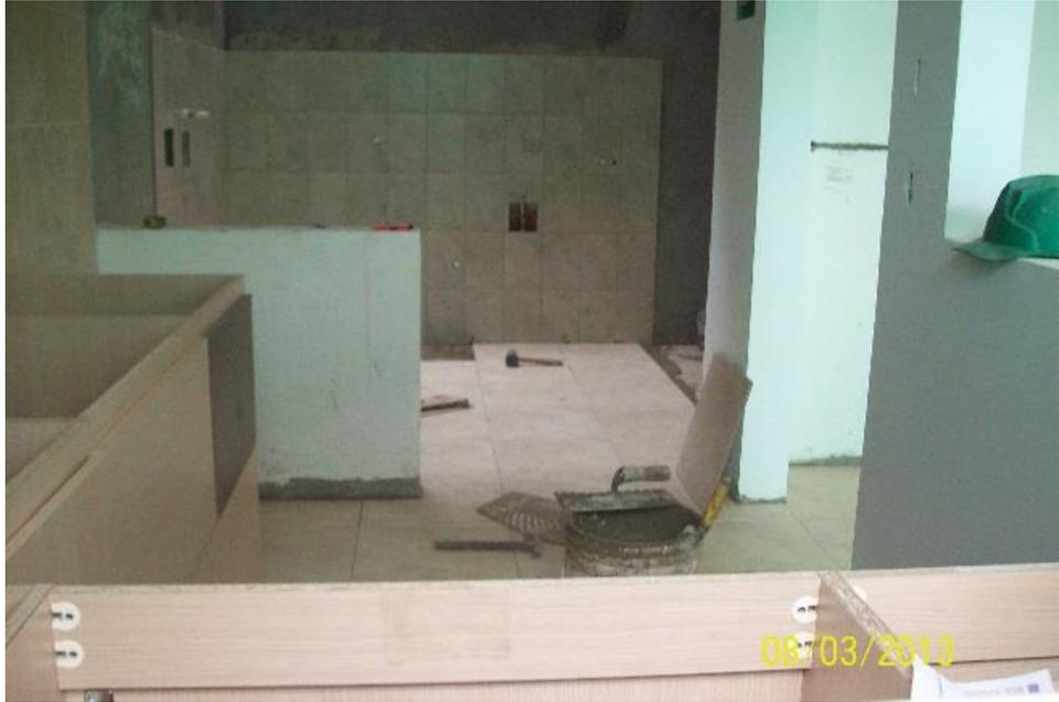
**Figura No. 88: enchape de muros**
