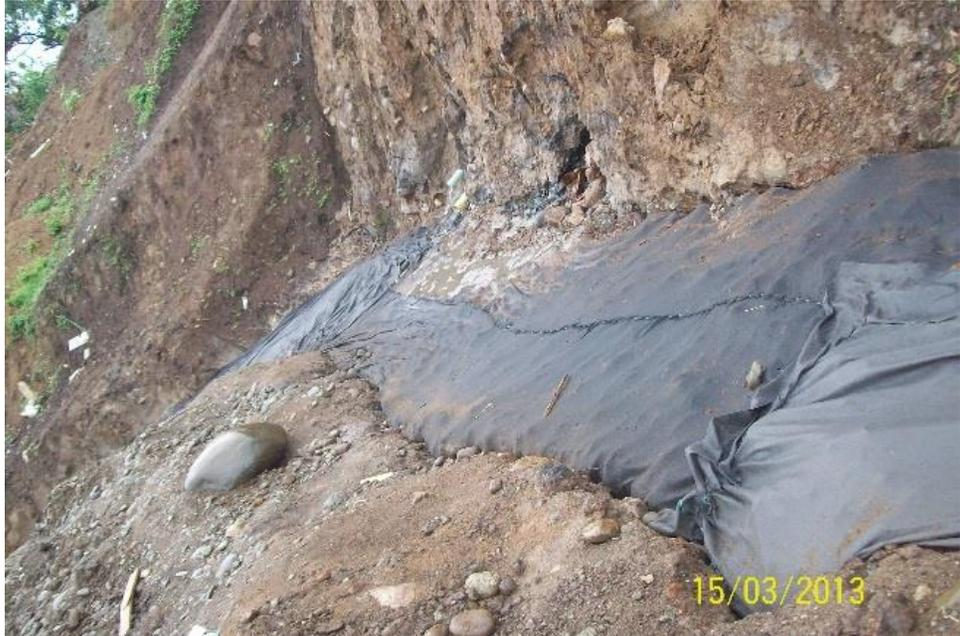
**Figura No. 137: geotextil cosido**
