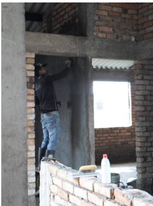
**Figura No. 81: repello de muros**
