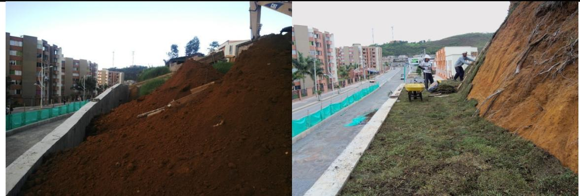
IMÁGENES No. 80. LLENO CON MATERIAL LIMO ARCILLOSO ENTRE EL MURO Y EL TALUD Y EMPRADIZADO.
