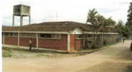
VISTA NOR-OCCIDENTAL-CONSULTA EXTERNA
