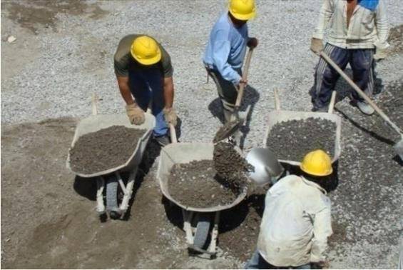
**Figura 26. Buggis para agregados**
