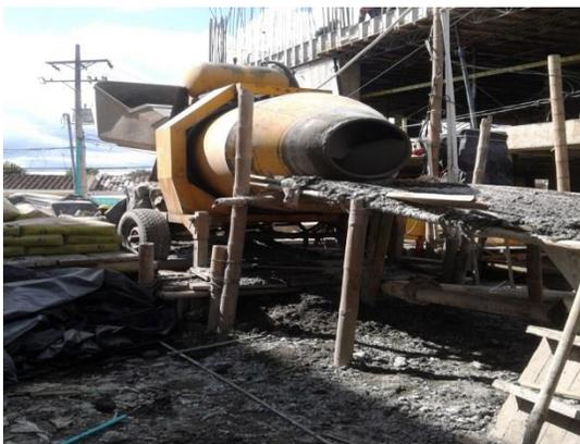
**Figura 53. Mezcladora de concreto**
