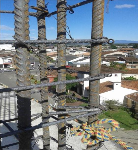
**Figura 42. Acero transversal estribos**
