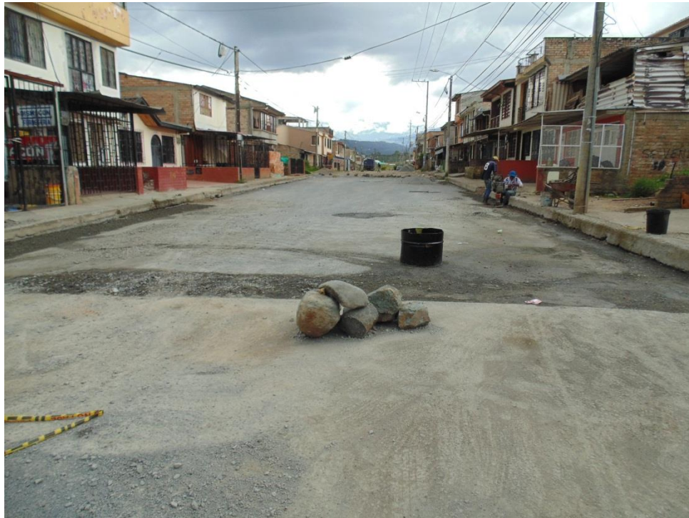
Figura 6.16 Base compactada
