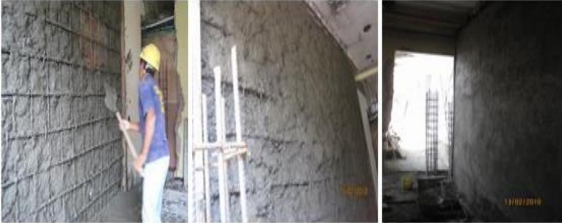
**Fig.52 Mortero estructural pantalla**
