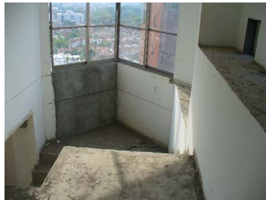
Escalera Pent House
