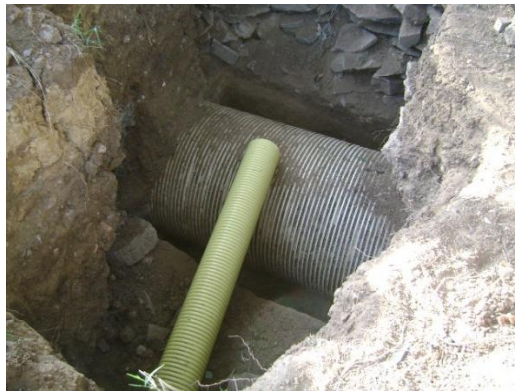
Figura 57. Empalme al colector principal
