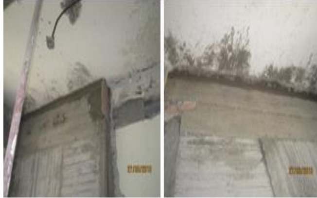
Fig.22 mortero 1:1 o Dray paking
