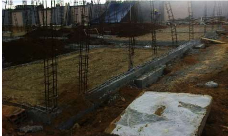
FIGURA No. 35 Relleno – sub base.
